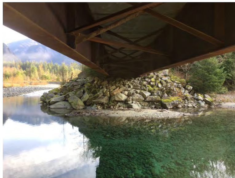
Left Bank Abutment when facing downstream
