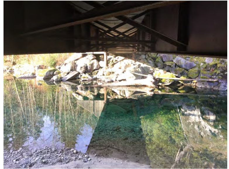
Right Bank Abutment when facing downstream
